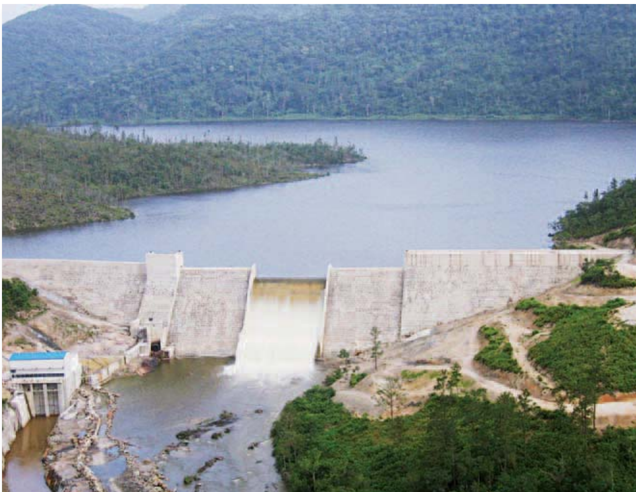
The Chalillo hydroelectric facility in Belize considerably minimized the impact of flood waters in San Ignacio after heavy rains.
